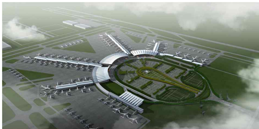
Northern Nanchang International Airport China
