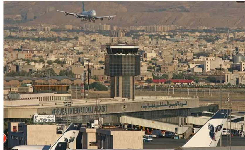
Mehrabad International Airport Iran
